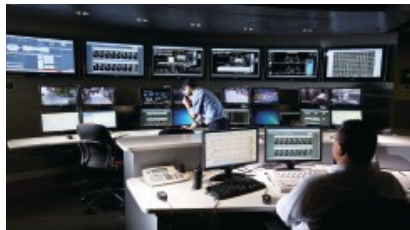
command and control center
